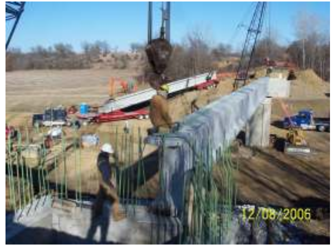
One beam is set and the next one arrives.
