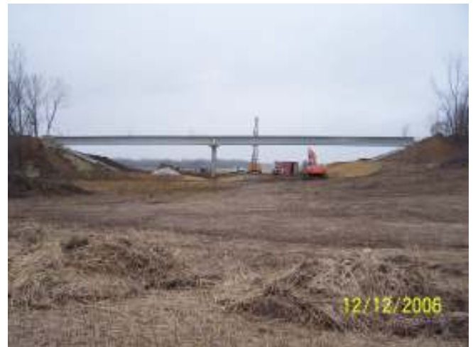
A side view as will be seen from the new highway.
