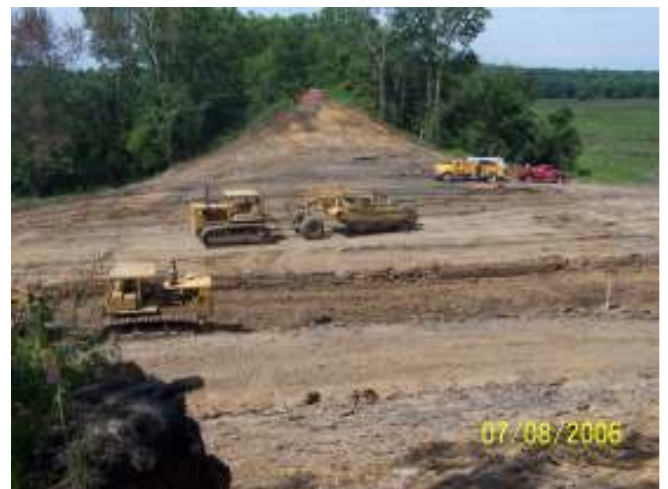
Contractor removes the trail & old RR fill
